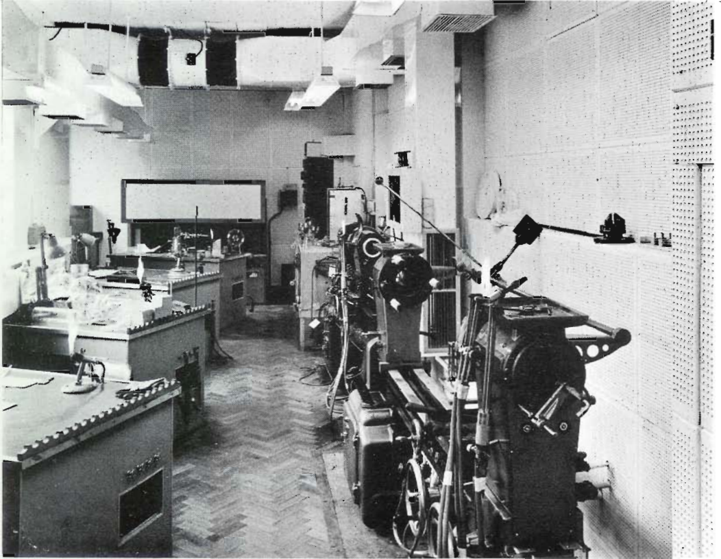
Photograph of Ducting System B
